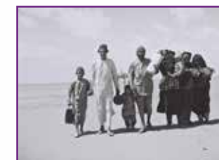
Courtesy of GPO, Zoltan Kluger, 1949
