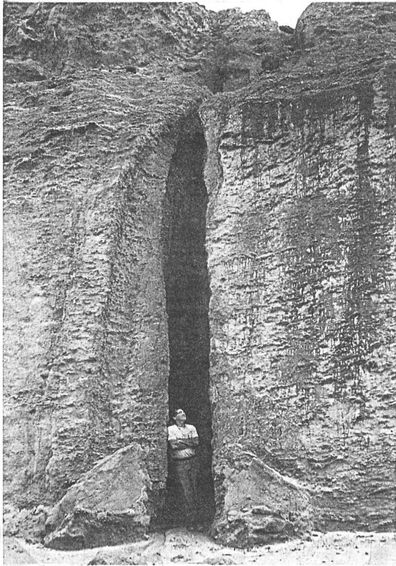
Fig. 8. A cylindrical scour pipe.
