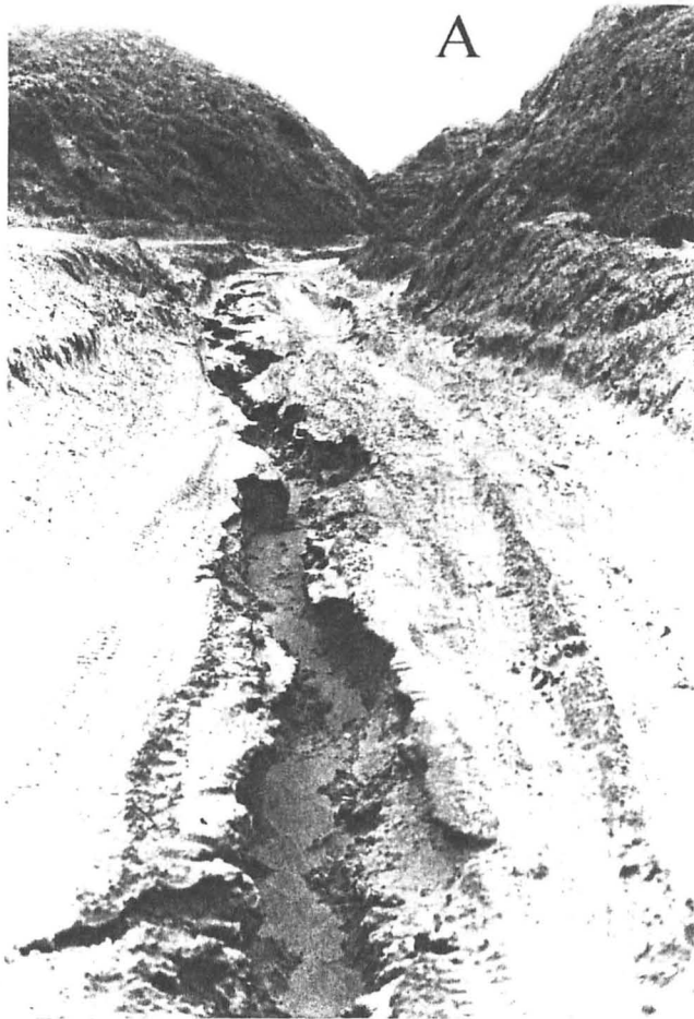
Fig. 22. A. Heavy erosion of a beachward descending road excavated at right angle to the cliff. ← B. Back-cutting erosion of the road in A creates badlands and gorges back of the kurkar ridge.
