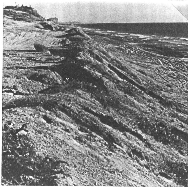
Fig. 29. A. Artificial talus, heavily scoured by rills subjected to rapid runoff gullyng. B. Talus was completely removed by wave swash.
