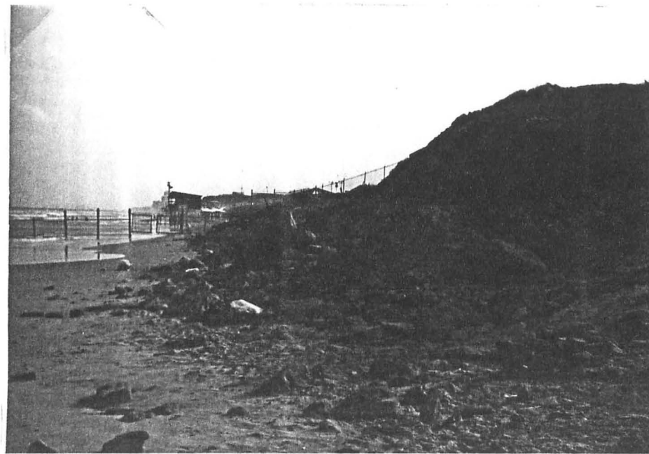
Fig. 29. A. Artificial talus, heavily scoured by rills subjected to rapid runoff gullyng. B. Talus was completely removed by wave swash.
