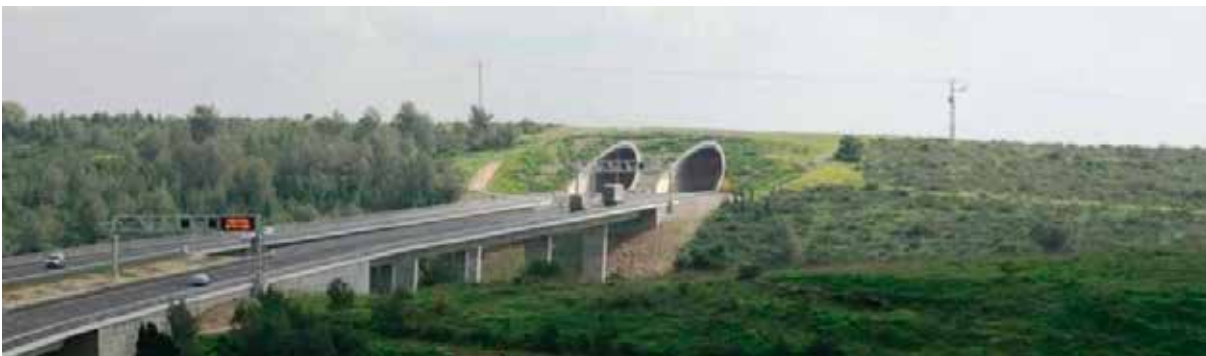
Monitoring programs that are conducted at each of these locations have shown heavy usage of these overpasses by wildlife. Photos: Dotan Rotem, NPA
