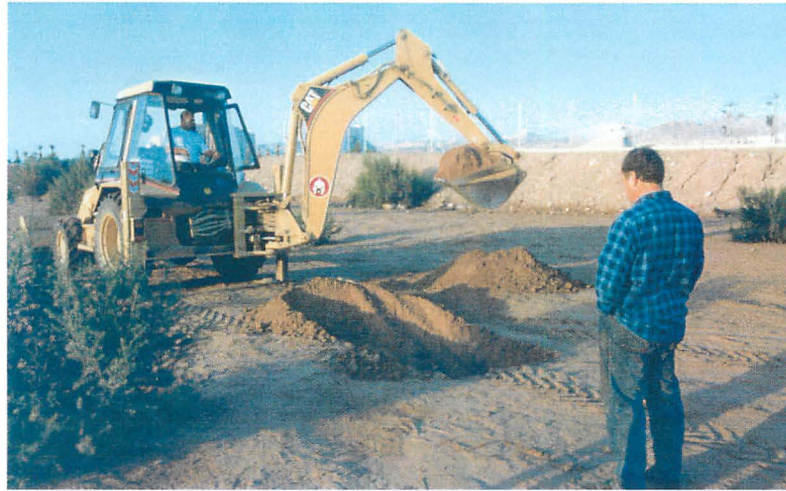
Figure 6.6. Trenching site C with a backhoe.
