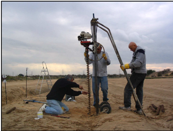
FIGURE 2.1: A drilling team preparing the installation of a ceramic cup.
