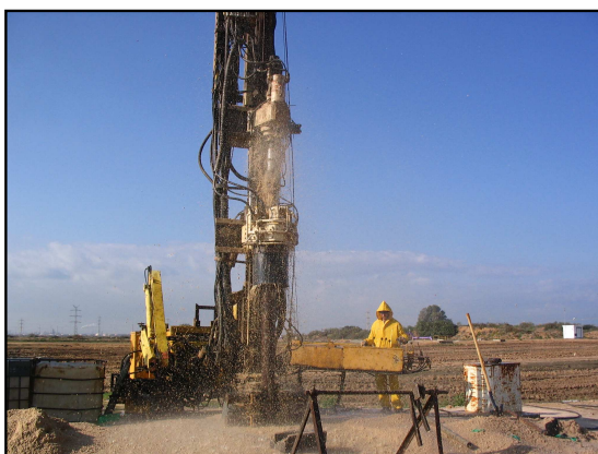
FIGURE 2.7: Drilling wells T/283, T/284 and T/285, using a dual system drilling instrument. The cuttings are removed from the borehole by compressed air.
