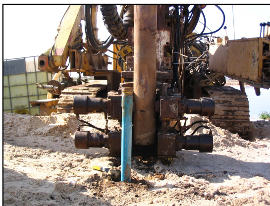
FIGURE 2.8: Installation of a 2" diameter PVC tube at the end of the drilling.
