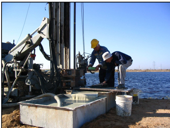
FIGURE 2.5: Drilling of wells T/281, T/282 using a rotary drill with drilling mud.
