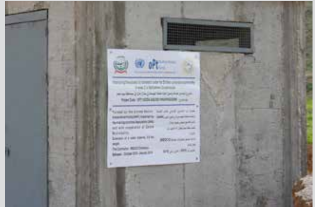
A pumping station, part of the water infrastructure established in the Nature Reserve by the United Nations agency UNHF and the Arab Fund for Development AAA
