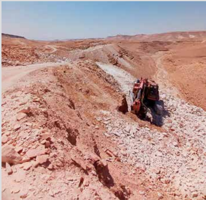
Quarrying along the route of Nachal Arugot
