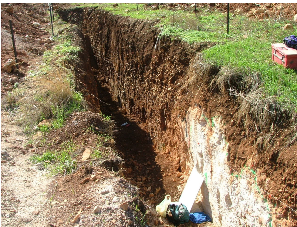
Fig. 8 – The transition zone (White color – Adulam Formation; Brown color – colluvial and alluvial sediments)
