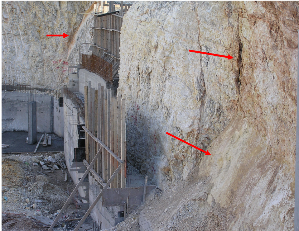
Fig. 6 – Exposure of the Nesher fault plane in a foundation pit of a building in the junction between Oskar Shindler road and Mendel Zinger St.
