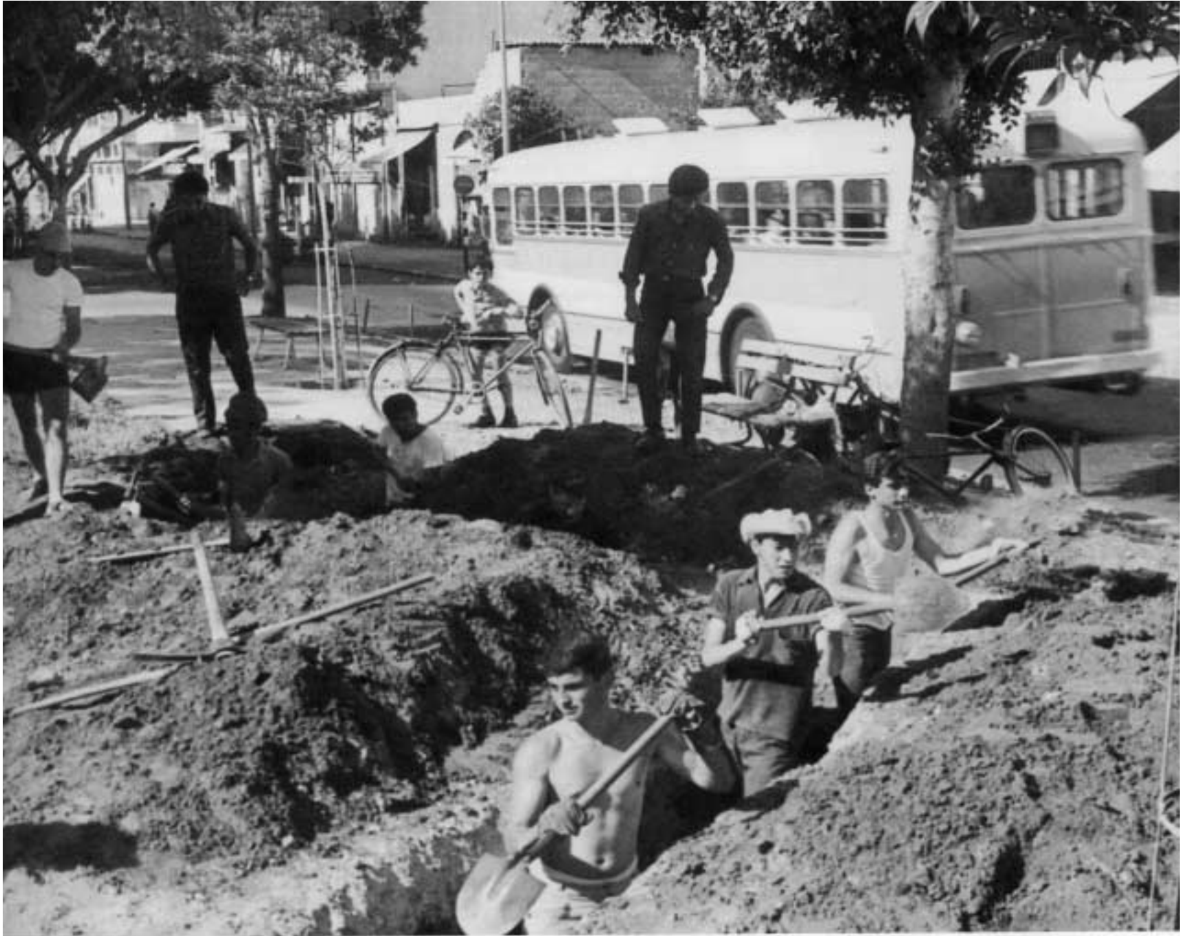
High school students digging air raid trenches in a Tel Aviv suburb (May 1967) in view of Arab calls to annihilate Israel on the eve of the Six Day War
