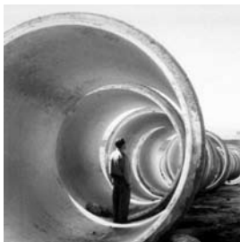
Concrete pipe section (108" diameter) of the National Water Carrier
