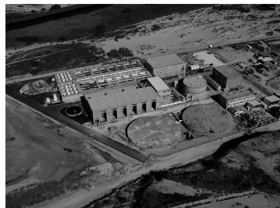
Fig. 4. 30 million m 3 /year Palmachim plant.
