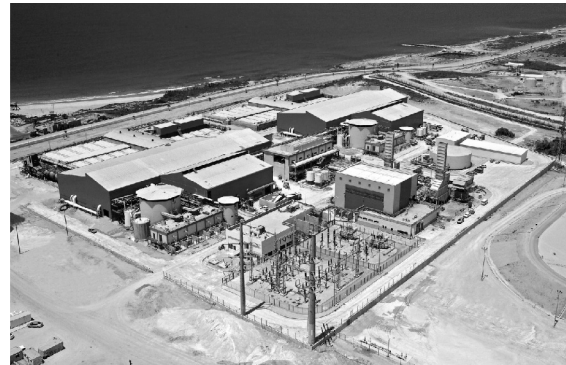
Fig. 3. 100 million m 3 /year Ashkelon plant.
