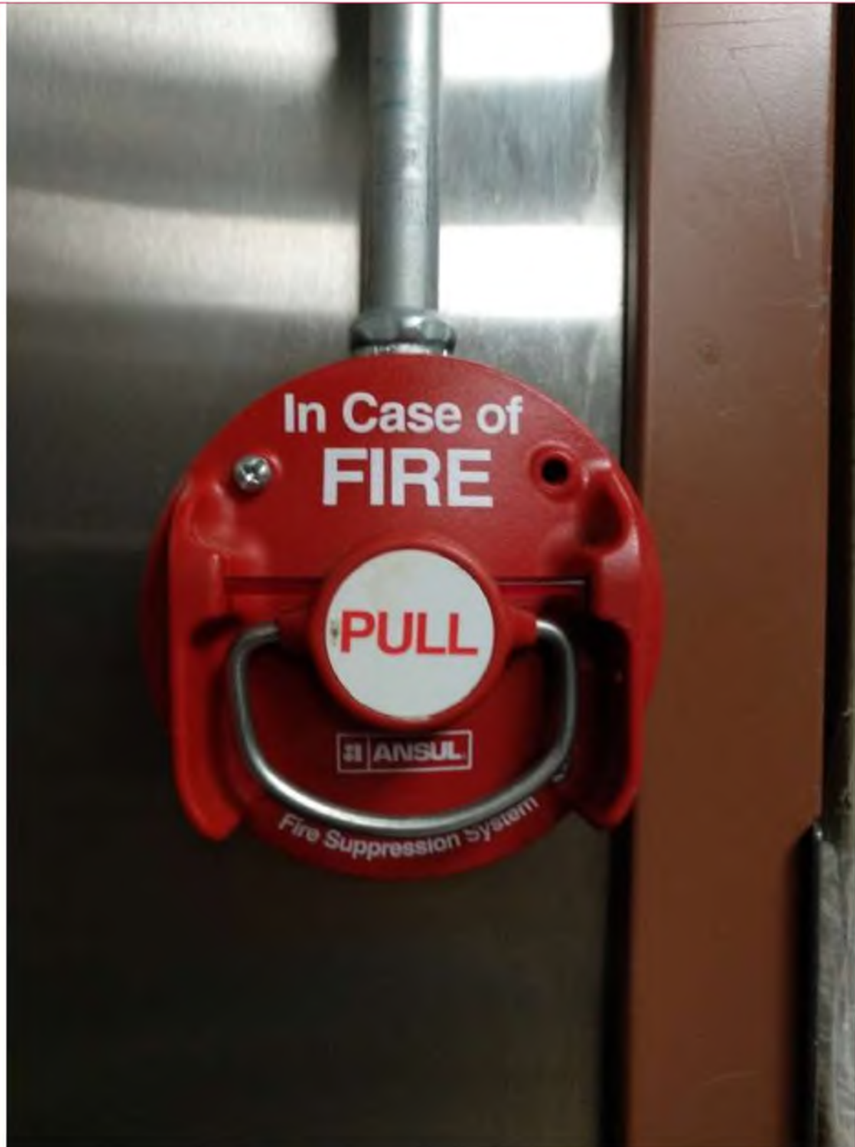
Figure 4: Suppression manual pull activating system.
