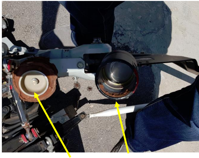
Red damper housing and separated elastomeric material
