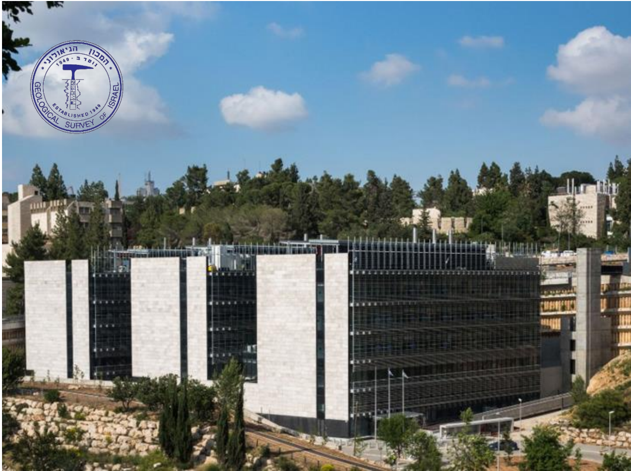
Fig. 2. The new Geological Survey of Israel building at Givat Ram, Jerusalem.
